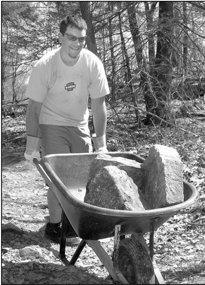
Most Blue Hills trail projects involve moving around lots of rocks. This load was headed for a project along Base Path. Photo by Joe Sloane
